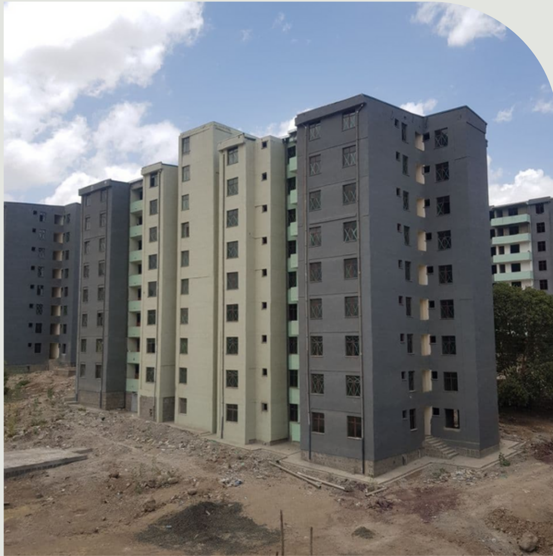
Housing Apartment project
